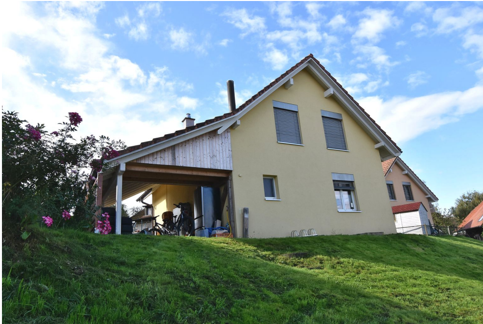
Photo N°5 Façade Nord (talus)
