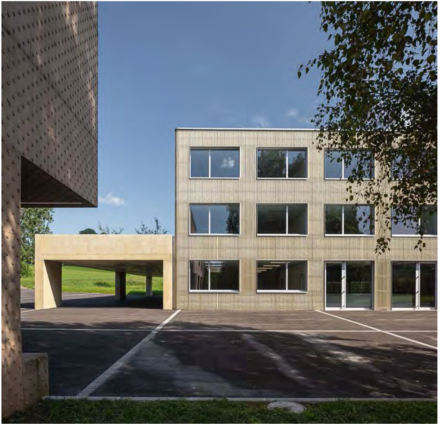
façade sud – angle enogone
